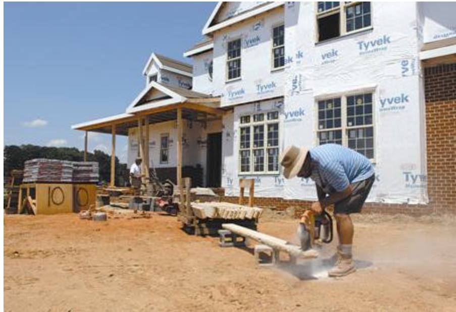
Ken Koons/Staff Photo Workers build a house in the Clover Meadow subdivision at the corner of Md. 91 and Deer Park Road.
